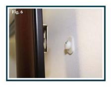
If you need to remove markers from the wall, grip the markers with pliers. Pull towards the ceiling at a 45° angle. For more information or a video demo on Level-Lock, visit www.level-lock.com.
